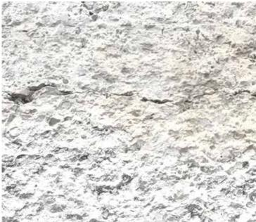
Its texture, thickness, crack-bridging capacity and color (light grey) have kept the original appearance of the facade.
