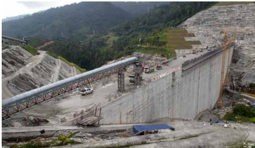
Figure 1.2.1: RCC dam construction
