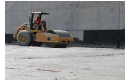
Figure 5.6.1: Compacting of RCC with a vibratory roller
