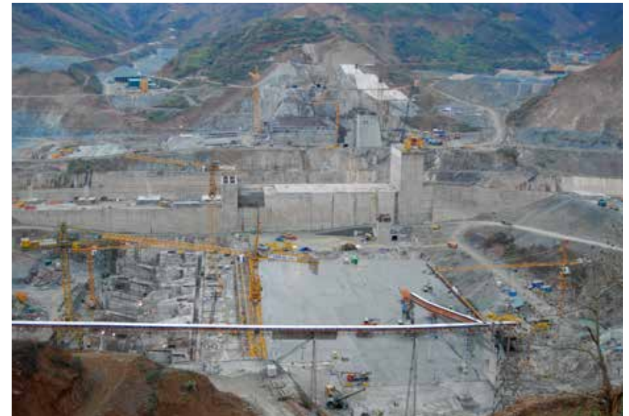
Figure 6.2.1: Surface preparation prior to RCC placement
