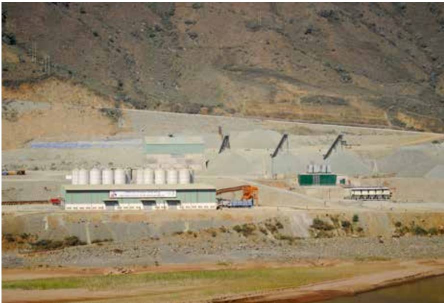
Figure 6.4.1: An aggregates plant near a dam site in Vietnam
