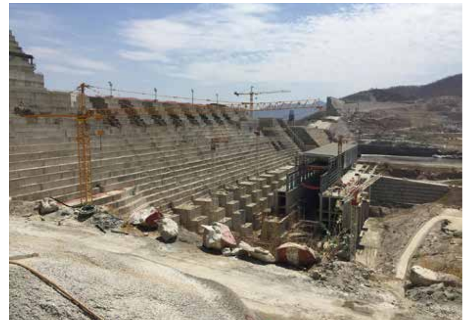
Figure 4.1.1: A RCC dam under construction
