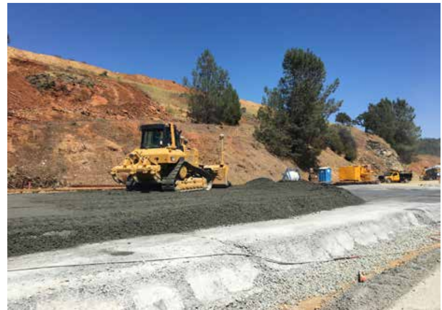
Figure 3.2.2.2: RCC spreading
