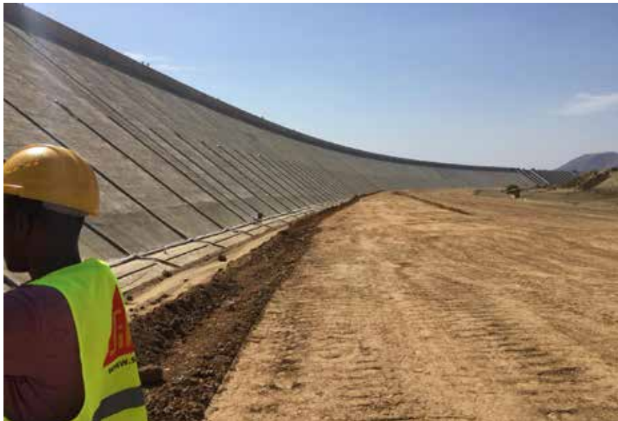
Figure 6.1.1: A saddle dam under construction in Africa
