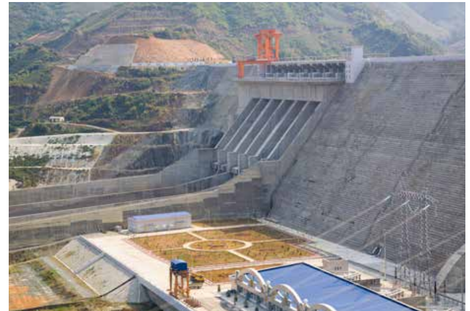
Figure 6.5.1: A spillway included in the RCC dam body
