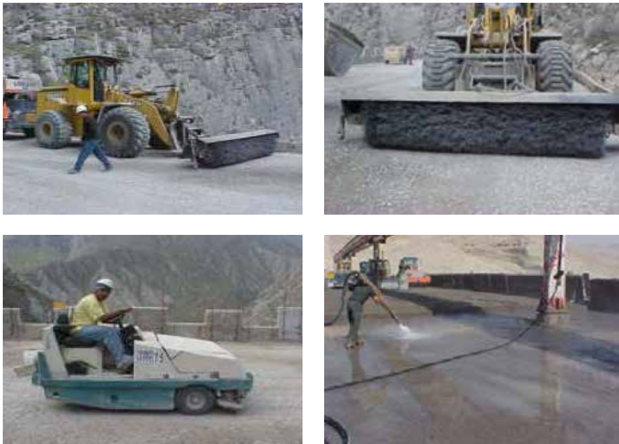
Figure 5.7.1: Cleaning methods of layer surfaces
