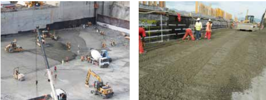
Figure 5.5.1: Placing and spreading operations
