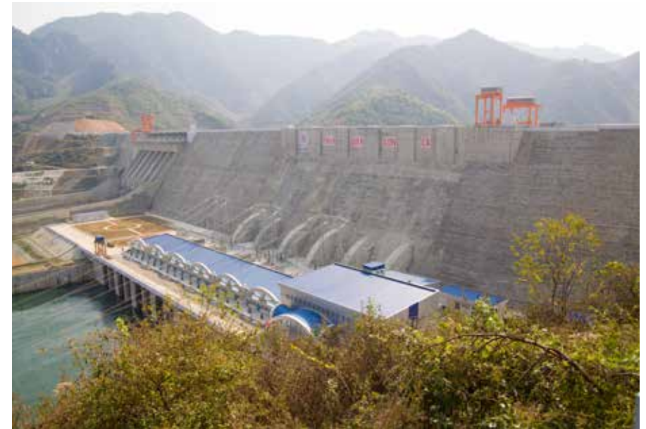
Figure 3.2.1.1: A completed RCC dam
