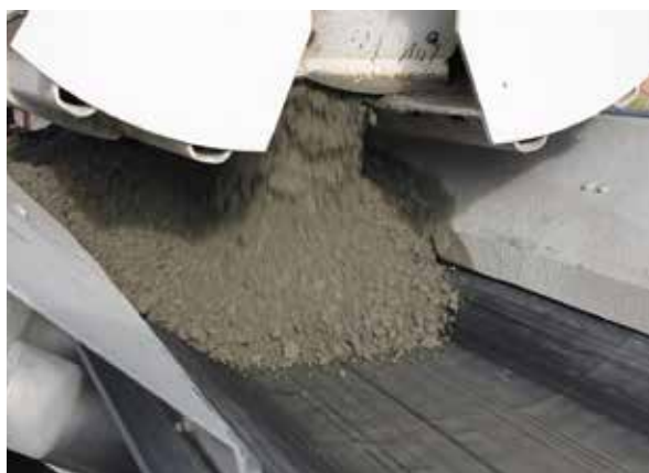
Figure 5.3.1: Production of Roller-Compacted Concrete
