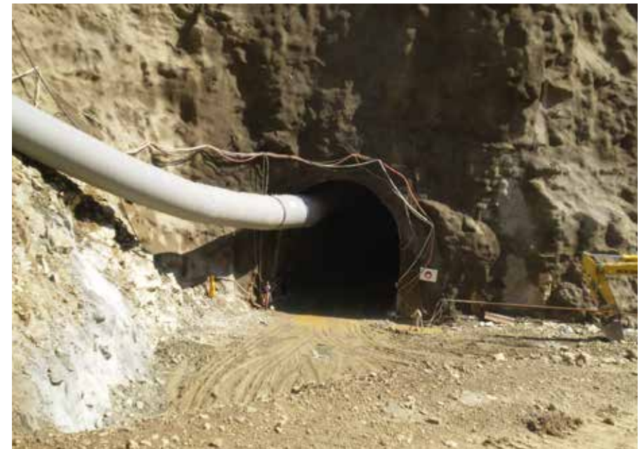
Figure 5.10.1: A gallery under construction at a RCC dam site
