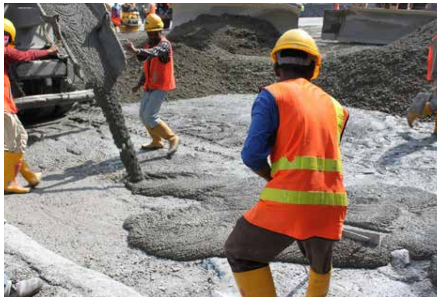
Figure 5.7.2.1: Laying and spreading of bedding mortar
