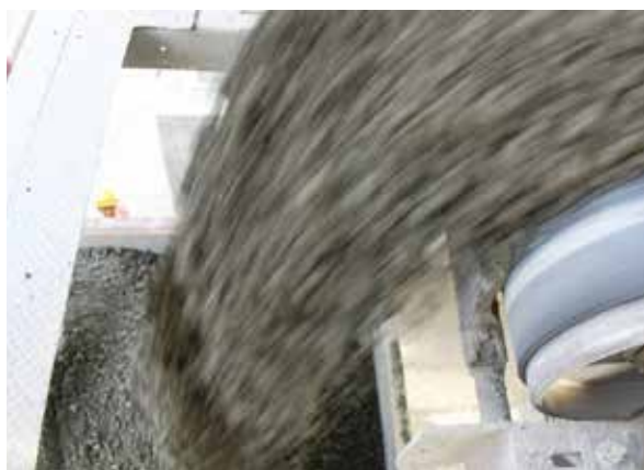
Figure 5.3.2: RCC discharged into a truck from the plant
