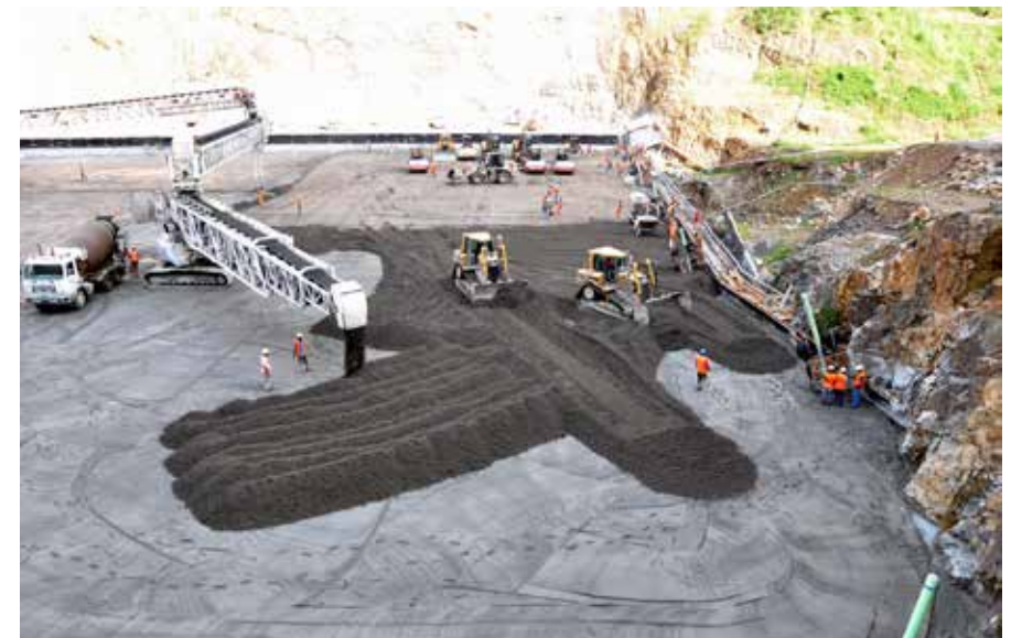
Figure 1.1.1: RCC spreading and compacting with dozers
