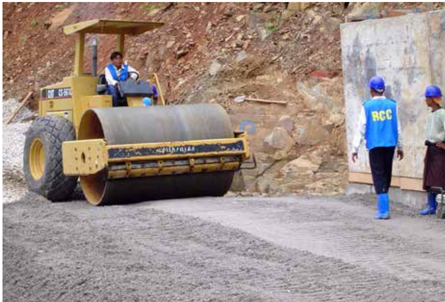
Figure 3.1.1: The RCC under compaction
