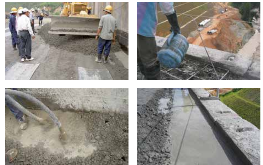
Figure 5.9.1: GERCC placement phases
