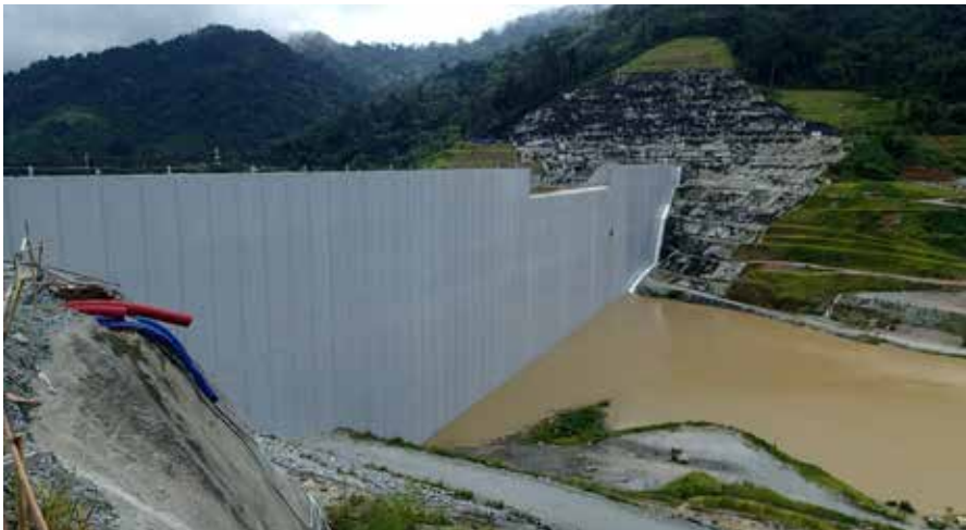
Figure 5.1.1: A completed RCC dam in the south of Asia
