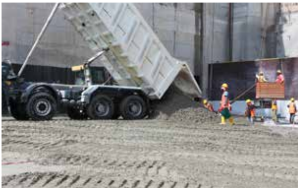
Figure 5.4.2.1: A truck unloads RCC at dam site
