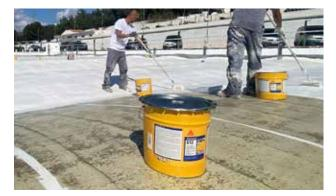
Finally, for the roof waterproofing, 12 tons of Sikalastic<sup>®</sup>-612 was sprayed applied. It is a single-component polyurethane membrane, applied cold, with technology activated by humidity, cold applied.
