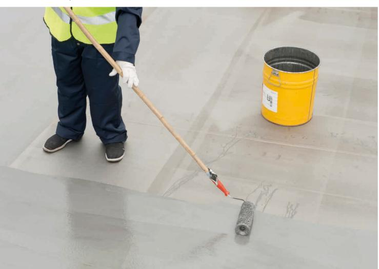
SikaCor® HM Mastic is the waterproofing layer. Its performance in varying trials greatly exceeds the standards. In addition, it is a good carrier of the hot-melt adhesive used as part of the system.
