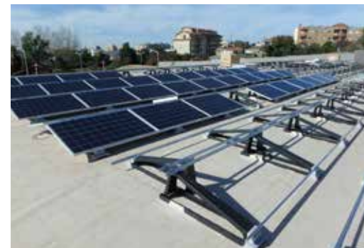
Installation in progress
