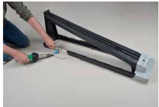
Hot-air welding of a Sika® SolarClick flange
