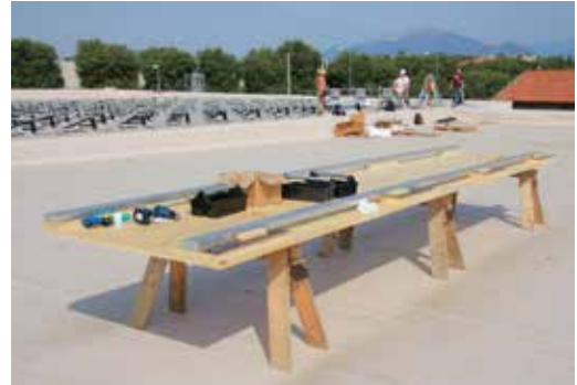
Preparation of system components on a workbench
