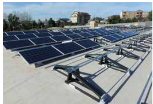
Installation in progress
