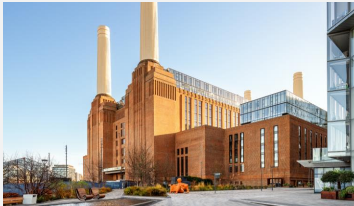
Battersea Power Station, London (UK)
