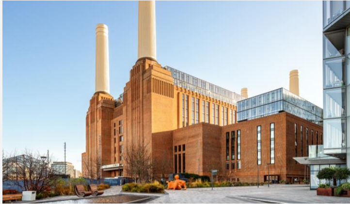
Battersea Power Station, London (UK)
