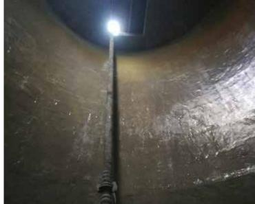
Sikagard<sup>®</sup> P 770 primer was applied by roller, followed by two coats of Sikagard<sup>®</sup> M 790 top coat in grey, applied by roller on consecutive days. A hot air blower was used to remove any condensation on the concrete surface during the coating process.
