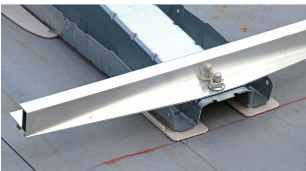
Mount positioning along the chalk lines
