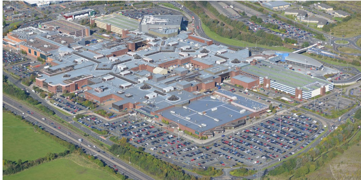
Shopping center MetroCentre (20,000 m 2 ), Gateshead, UK.
