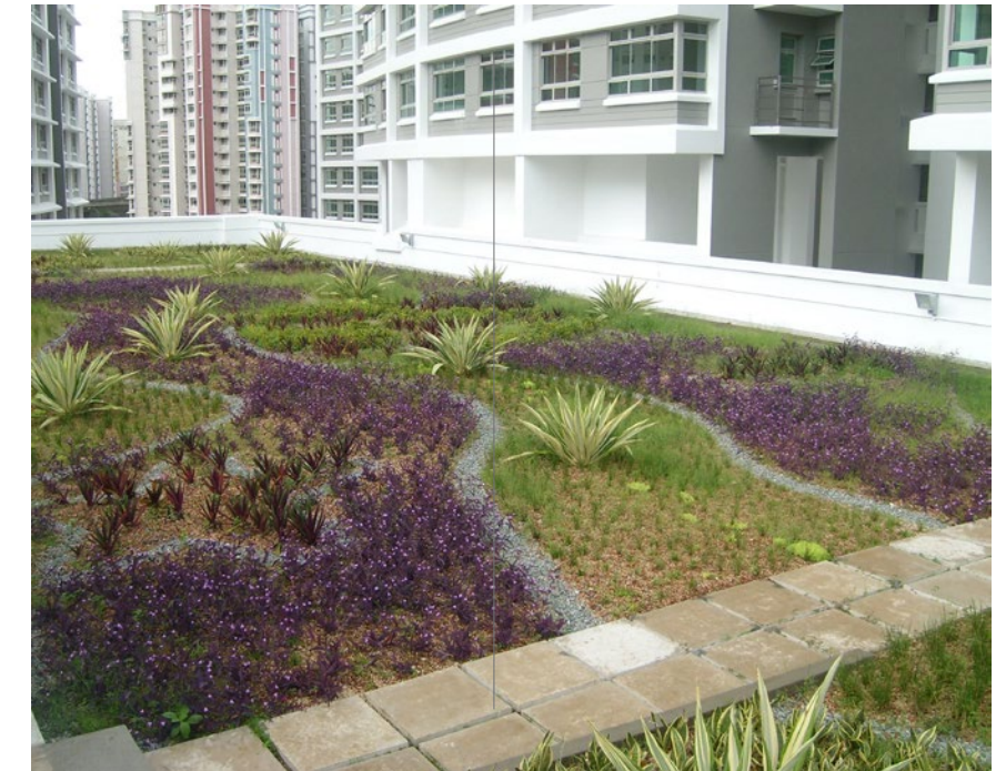
Sarnafil® Green Roof 2 for HDP Multi-Storey Carpark (public housing).
