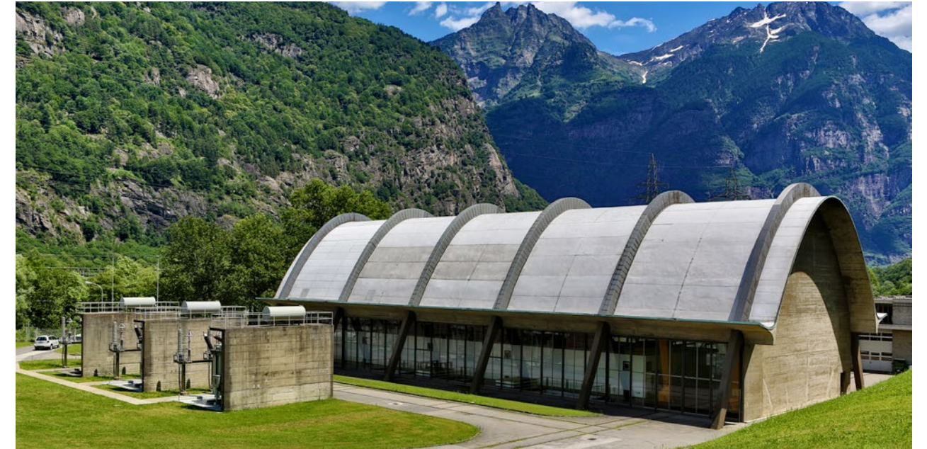
Hydroelectric power plant in Personico, Switzerland (installed 1976).
