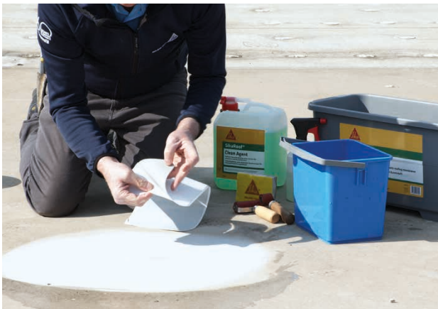
7. Remove of finger-lift release liner.
