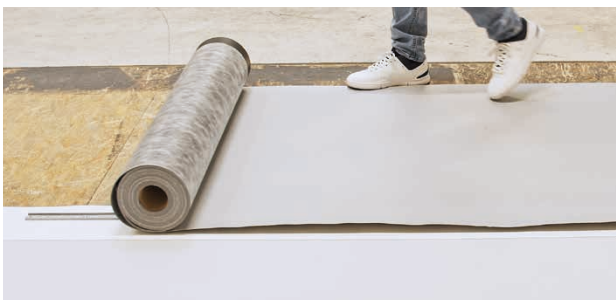
3. Roll-out of new Sarnafil® FPO roof waterproofing membrane.
