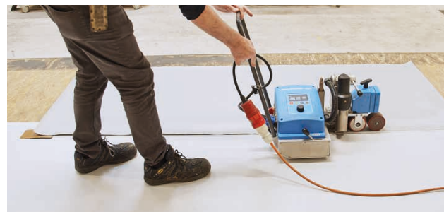
4. Automatic hot-air weld of Sarnafil® FPO membrane onto SikaRoof® Multitape.
