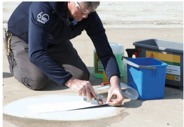
8. Attaching of SikaRoof® Multitape with pressure roller.
