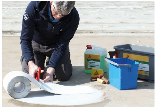
6. Cut SikaRoof® Multitape to the needed length.
