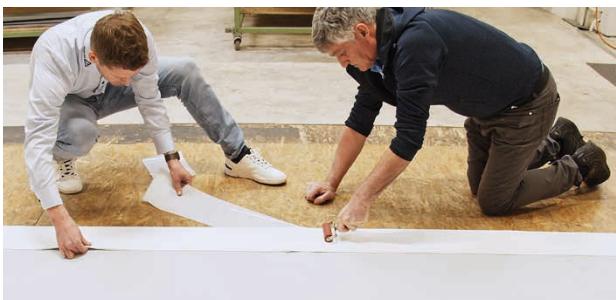
1. Installation of SikaRoof® Multitape on top of existing synthetic or bituminous roofing.
