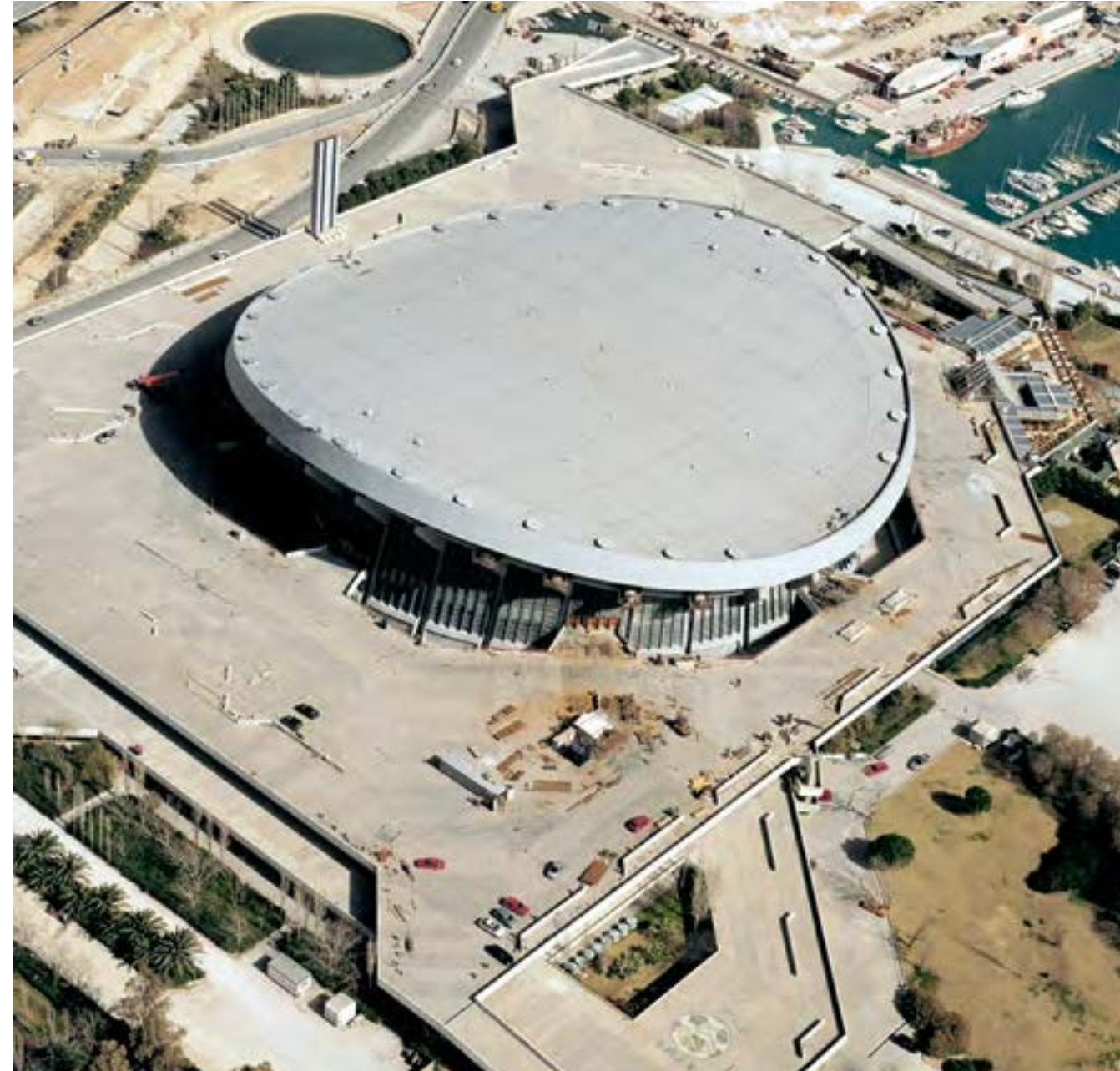
Project year: 2003 | Peace and Friendship (SEF) Stadium, Athens Palio Faliro, Greece Sarnafil® TS 77-15, RAL 7040
