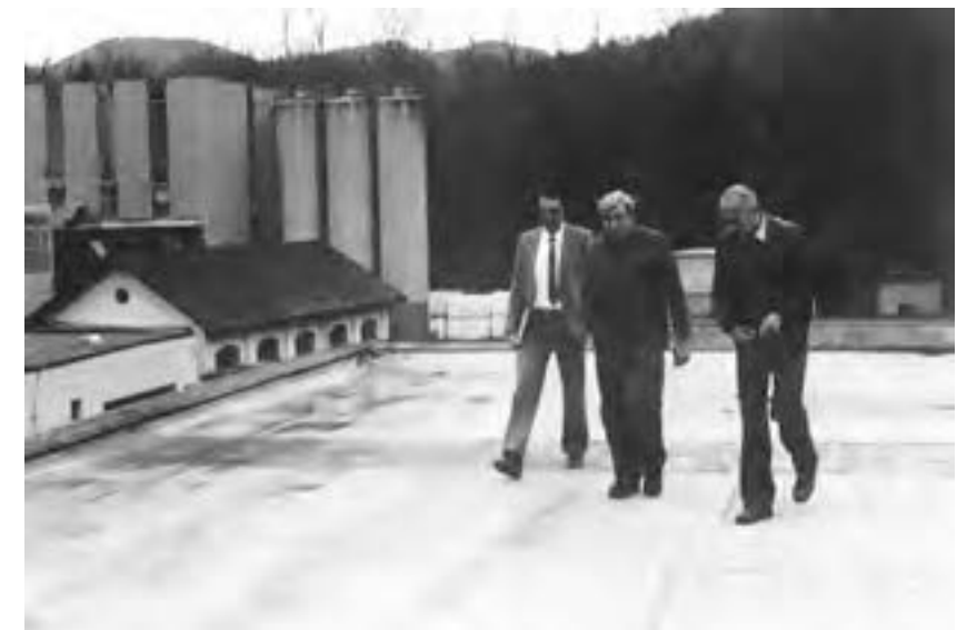
Project year: 1964 | Industrial building of Galban AG, Burgdorf, Switzerland Roof was renovated in 2010
