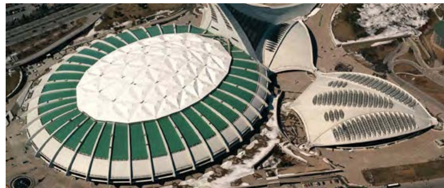
Project year: 2004 | Montreal Olympic Stadium, Montreal, Quebec, Canada Sarnafil® G 410-30, 120 mil membrane webster green
