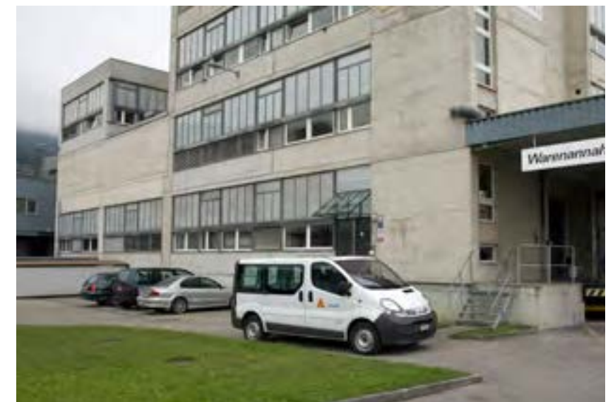
Project year: 1989 | The first Sarnafil® T project at Warehouse Sarnafil, Sarnen, Switzerland
