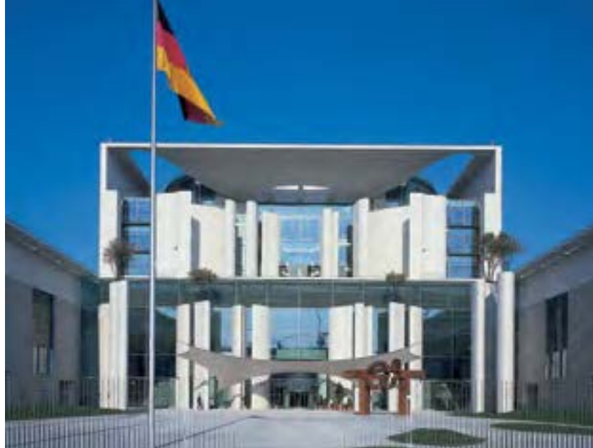
Project year: 2000 | Federal Chancellery, Berlin, Germany Sarnafil® TG 66-20
