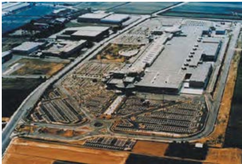
Project year: 1990 | Curno Shopping Center, Curno, Italy Sarnafil® G 442-15; Sarnafil® G 476-15; Sarnafil® G 476-20
