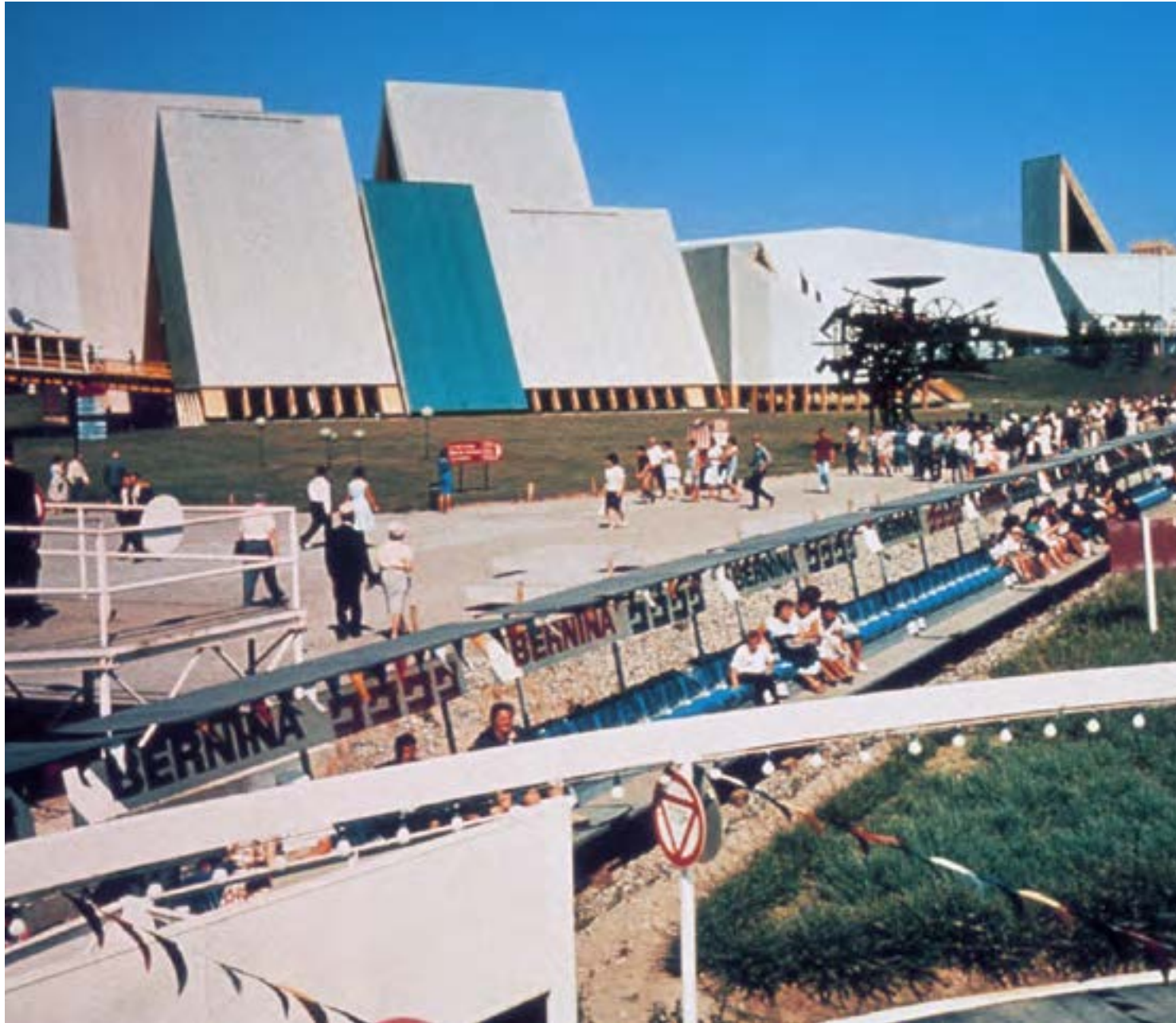
Project Expo 64 gave Sarnafil® the opportunity to waterproof a total of 42,000 m 2 roofs, including Swiss Path, Festival Hall, Military Pavilion and Monorail. This exposition introduced the Sarnafil® membrane to building professionals throughout the world.
