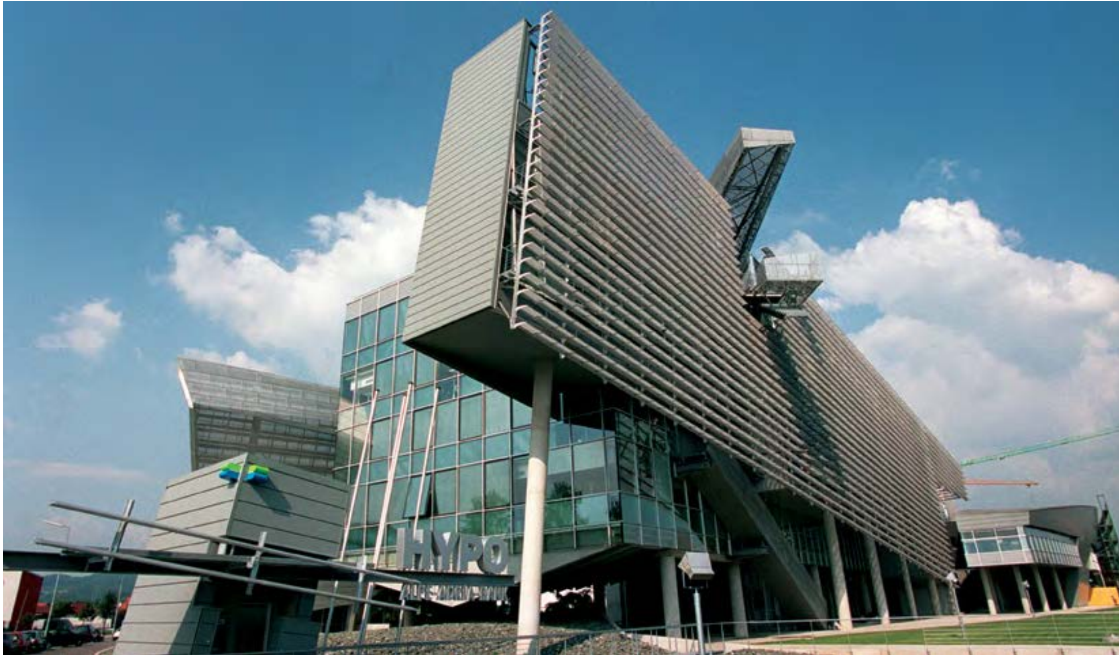
Project year: 1998 | Hypo Bank, Klagenfurt, Austria Sarnafil® G 442-15
