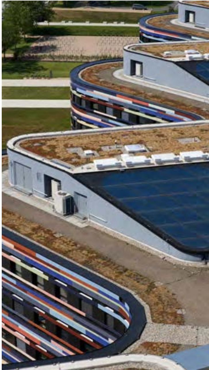
Project year: 2013 | Ministry of Urban Development and Environment Building, Hamburg, Germany Sarnafil® TG 66-20
