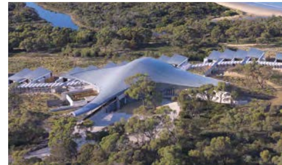
Project year: 2010 | The Saffire Resort Coles Bay Tasmania, Australia Sarnafil® G 410-15L Felt, (RAL 7031) blue grey
