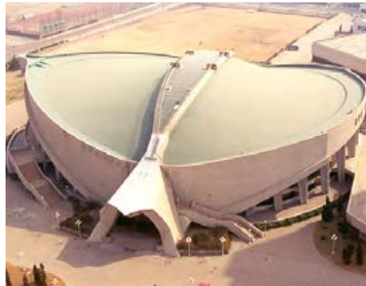
Project year: 1999 | Qindao Stadium, Qindao, China Sarnafil® 12F
