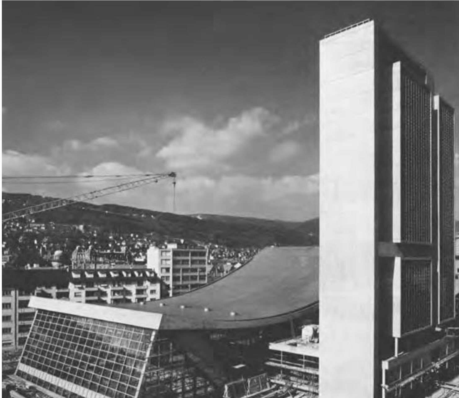
Project year: 1964 | Congress House / Swimming Hall, Biel, Switzerland Sarnafil® G 410-12; Sarnafil® G 410-18
