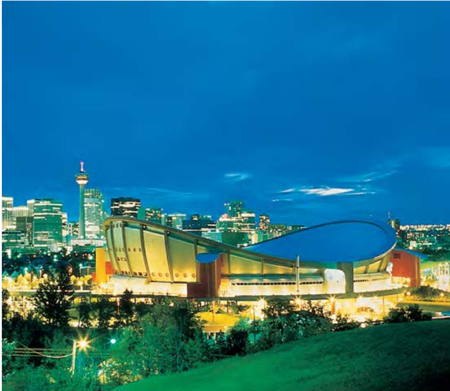
Project year: 1988 | Scotiabank Saddledome Arena, Calgary, Canada Sarnafil® G 410-12EL
