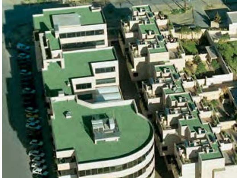
Project year: 1991 | Municipal Building Mustoles, Madrid, Spain Sarnafil® G 410-14, RAL 6011
