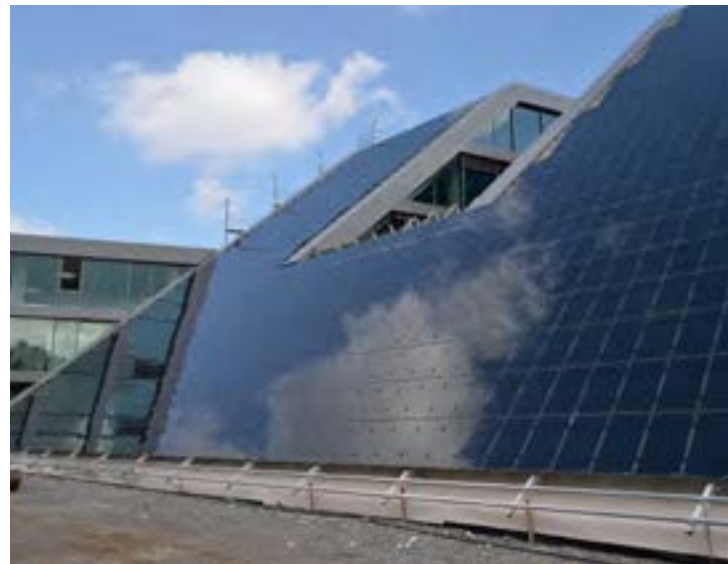
Project year: 2013 | Hahn und Kolb Administration and Logistic Center, Germany Sarnafil® TG 76 Felt, Sarnafil® TG 66 and SikaRoof® MTC 22
