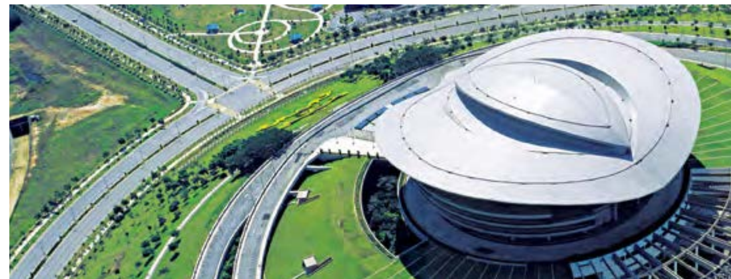
Project year: 2002 | Putrajaya Convention Centre, Putrajaya, Malaysia Sarnafil® S 327-15, Champagne colour
