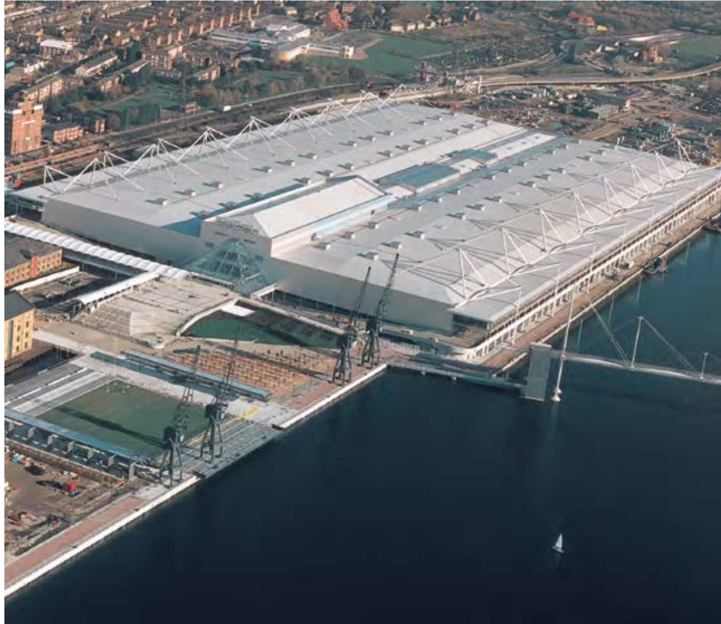
Project year: 2000 | ExCel Exhibition Centre, London, UK Sarnafil® S 327 and walkway plates
