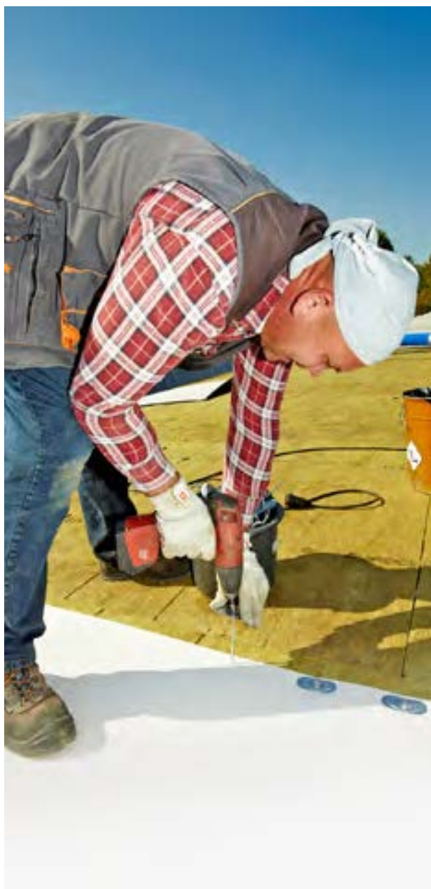
1989 | Sarnafast® spot fastening in overlapping mechanically fastened roof systems was introduced to resist wind uplift and for increased speed of installation.
