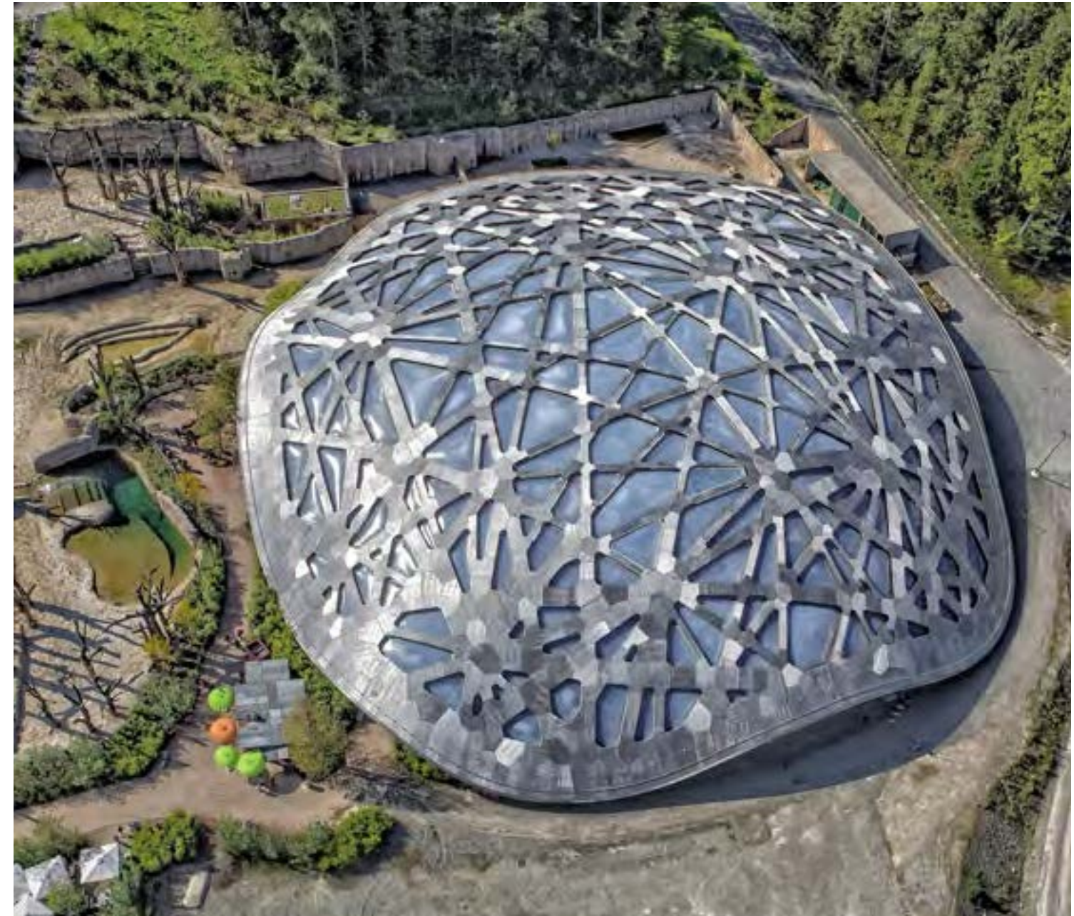
Project year: 2013 | Elephant House, Kaeng Krachan, Zoo Zürich, Switzerland Sarnafil® TG 76-18 Felt, RAL 7040, Sikalastic® 841.
