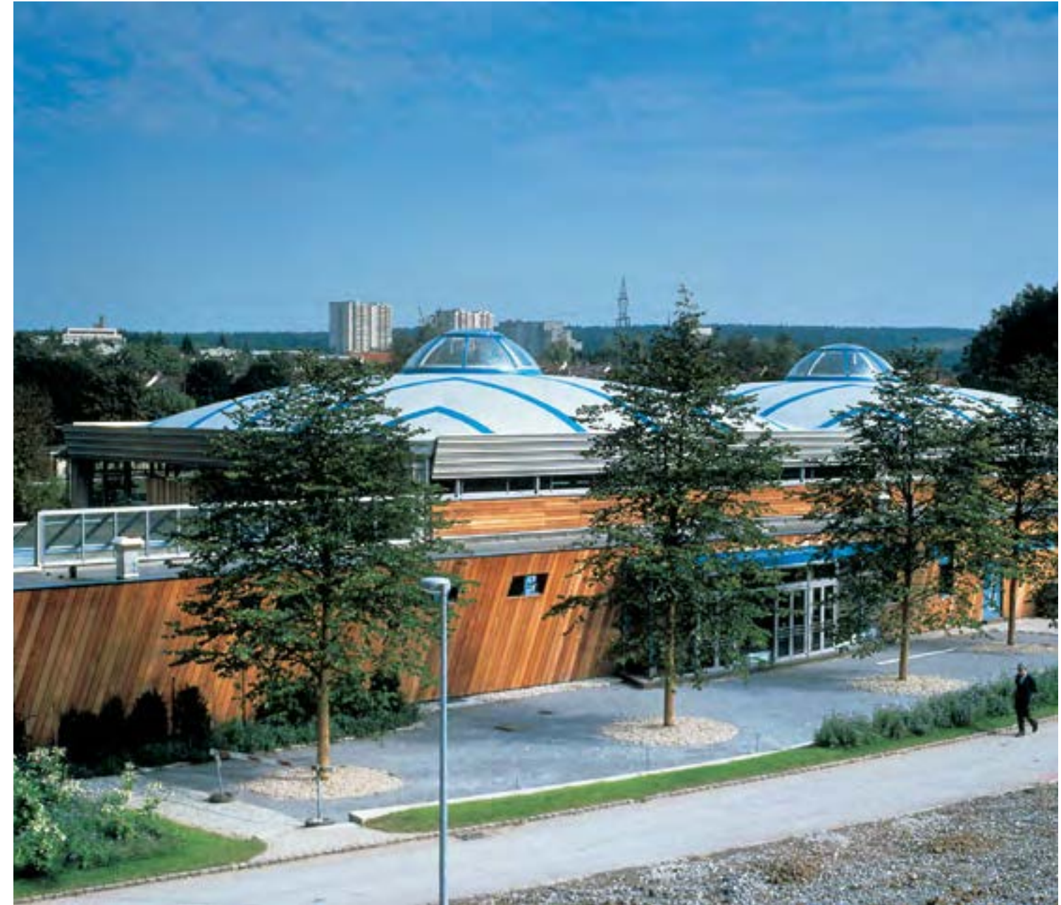
Project year: 1988 | Klosterseehalle, Sindelfingen, Germany Sarnafil® G 410-12EL
