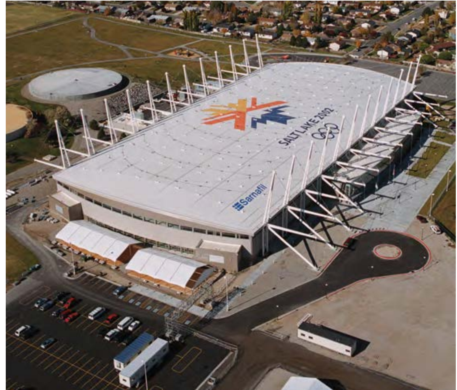
Project year: 2000 | Utah Olympic Oval Salt Lake City, Kearns, UT, USA Sarnafil® S 327; EnergySmart white and custom colour logo
