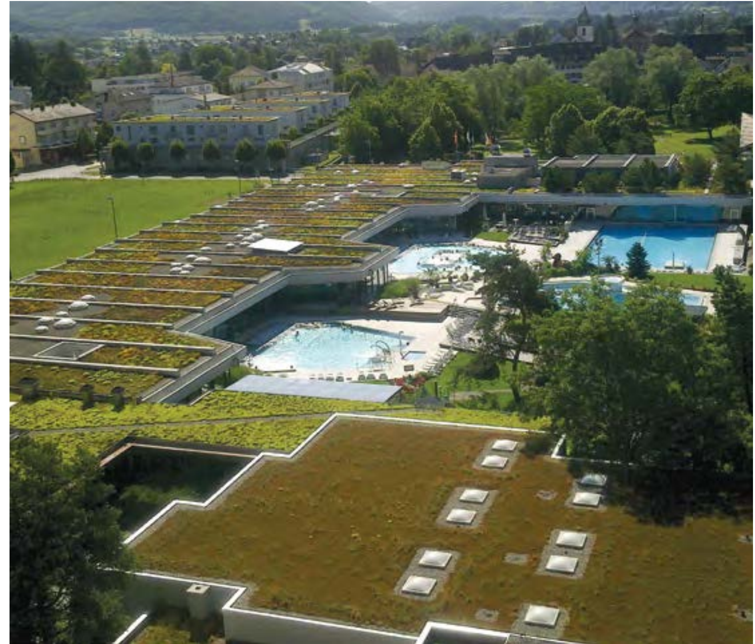
Project year: 1969 | The first project of green roof installation at Thermal Bath, Bad Zurzach, Switzerland
