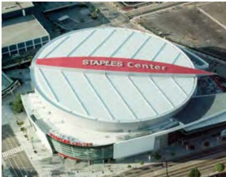
Project year: 1998 | Staples Center, Los Angeles, CA, USA Sarnafil® S 327, Sarnafil® G 410 custom matched "Staples Red" for backdrop of Logo
