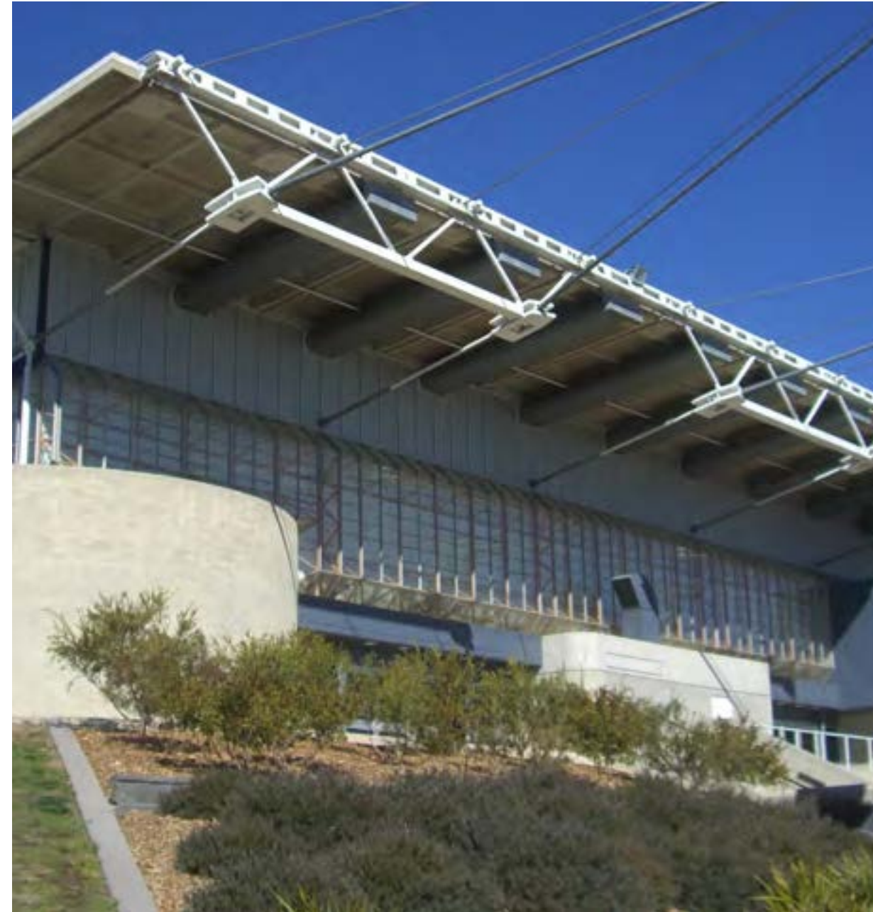
Project year: 1981 | Australian Institute of Sport AIS Arena Canberra, Australia
