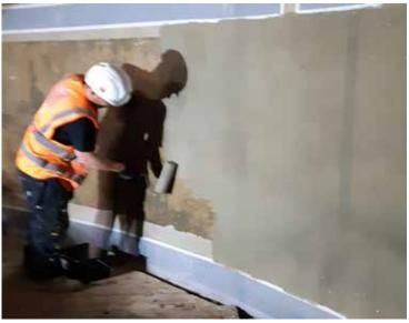
The surface below the gas zone was treated with a diluted solution of SikaLatex® to seal microcracks in the concrete. SikaEmaco® N 5200 was used to repair sections of failed concrete on the external walls of the digestor.
