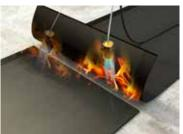
If a second layer is specified, it must be laid to straddle the overlap of the previous layer and must be bonded in complete adhesion. The burner flame must also heat the membrane already laid.
