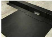
■ Proceed with the application of the first layer of the bituminous membrane, which cannot cover the drain area.
