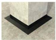
■ Cut another piece of the membrane enough to cover the entire corner angle. This must be done for all the corner joints. Then proceed with the application of the first layer of the bituminous membrane.
