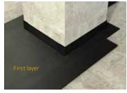
■ Apply again another piece of membrane on top of the fisrt layer, now on the opposite side of the corner. In this case, the overlapping should have an angle of 45°.
