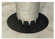
■ Cut another piece of membrane, same size as the first, and bond on the opposite direction. Then proceed with the application of the first layer of the bituminous membrane.
