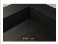
■ In case of a multilayer system, proceed with the application of the second layer following the same steps, but now starting on the opposite side of the corner.
