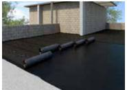
The overlaps must be sealed using other sealing product or by torch or welding.
