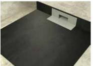
■ Cut and apply another piece of the membrane, enough to cover 15 cm higher than the size of the drain and more 10 cm on the top. Cut more two pieces of the membrane, enough to cover 10 cm of the top and the surface. Then apply on both sides of the drain.
