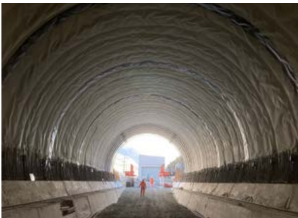
Mined Tunnel (drained) + Cross-passage, Switzerland, SikaProof®-200, 30,000 m 2
