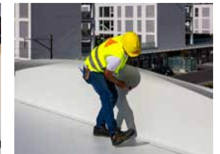
3. Attach the self-adhered membrane.
