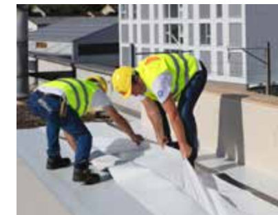
1. Position and remove Sarnafil® AT FSA P release liner.
