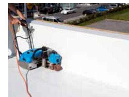
5. Complete the final hot air seam welding.
