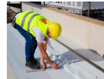
2. Mark the upper parapet edges.
