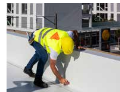
4. Press the membrane into place with a suitable roller
